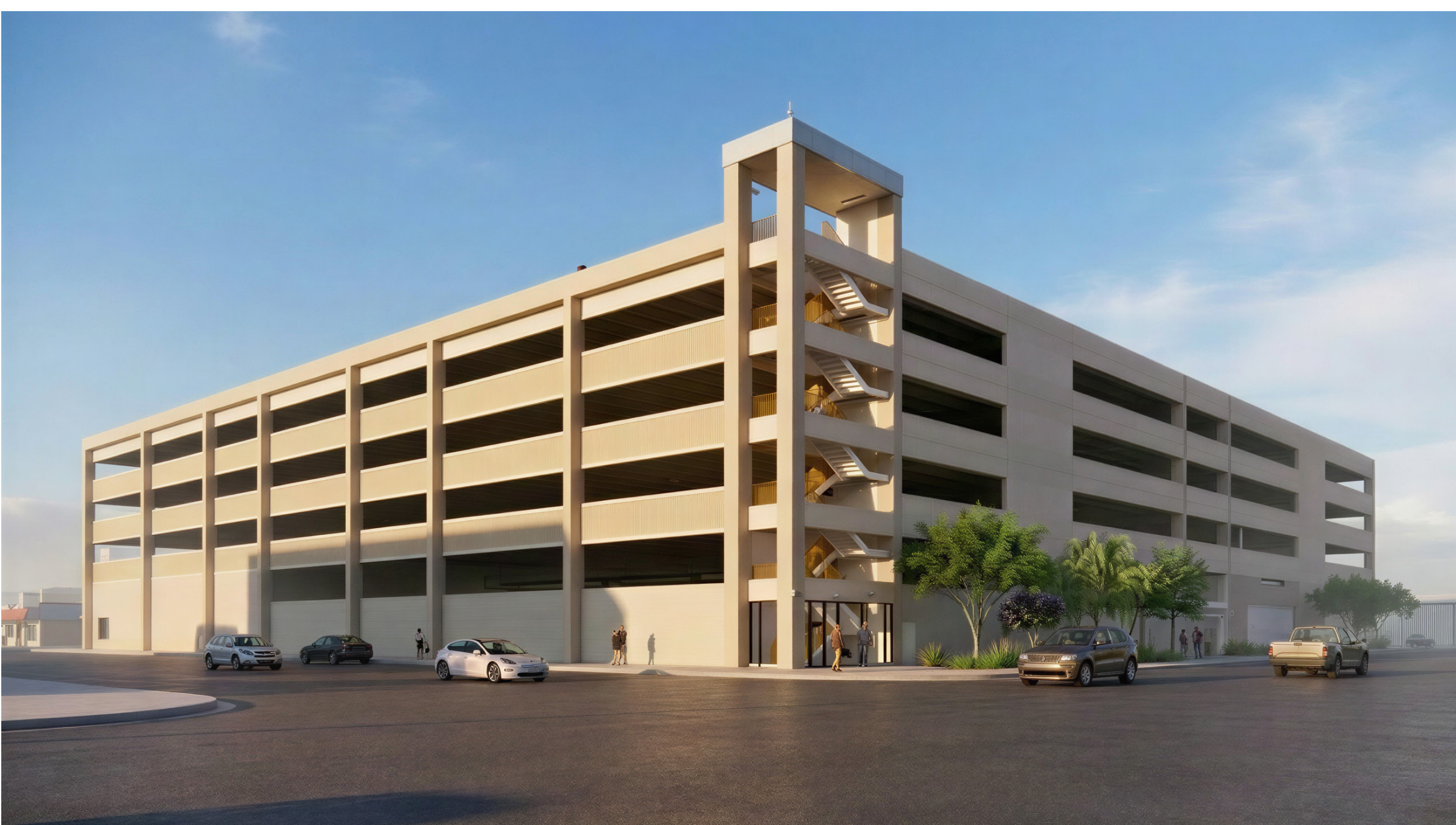
Parking Garage | Southeast Corner
