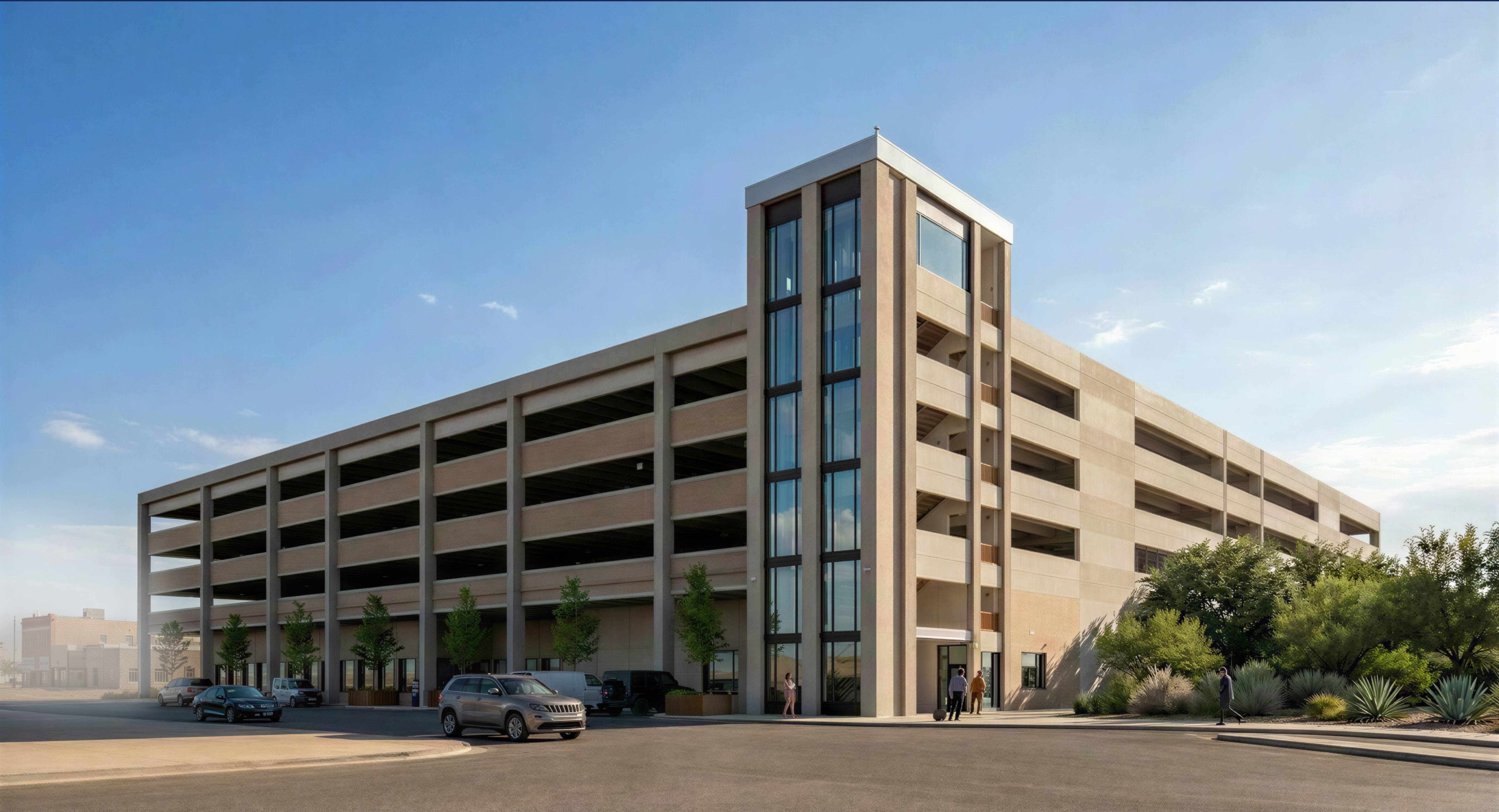
Parking Garage | Northwest Corner
